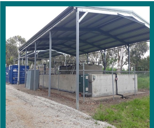
Coldstream leachate plant – the plant processes leachate liquid collected from the landfill for disposal into the sewer system. This is important to ensure that the liquid does not contaminate local groundwater and the surrounding environment.
