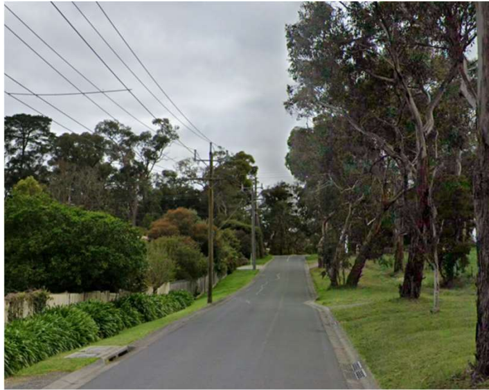
Similar type project: Fortune Avenue, Lilydale/Mt Evelyn 5m trafficable width with rollover kerb
